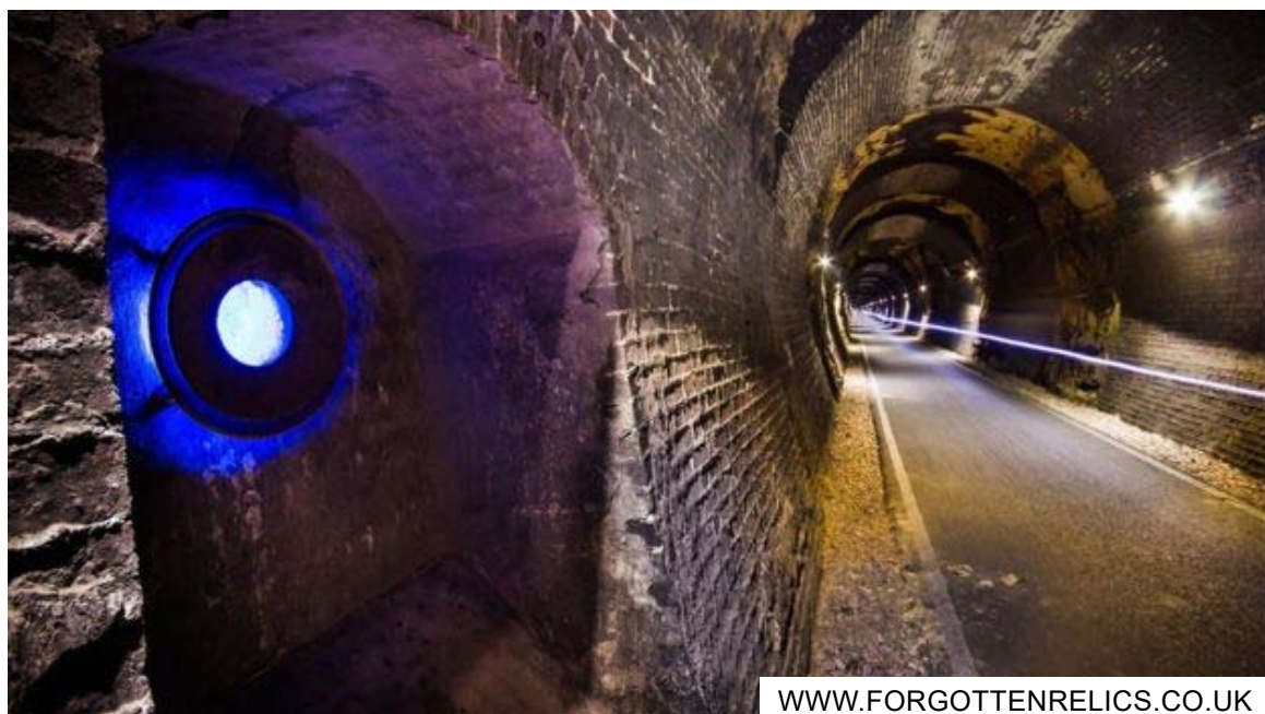
Combe Down tunnel after works
